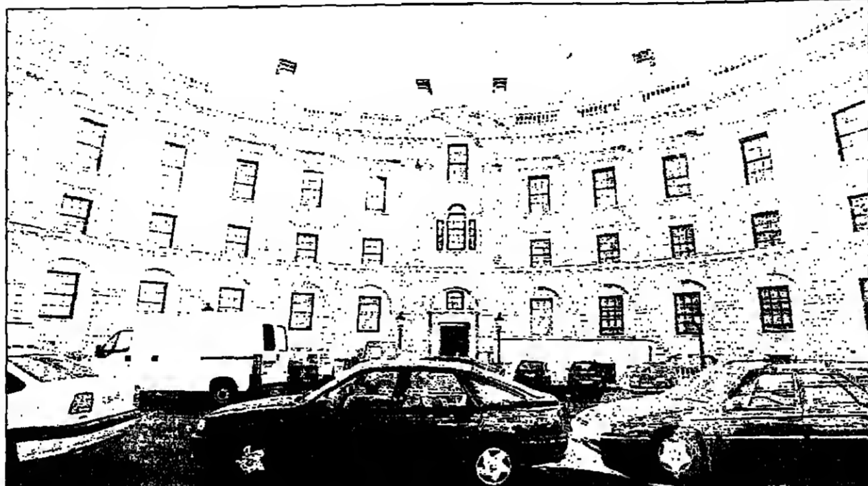
Whitehall link to Downing Street: the elegant circular courtyard where Treasury ministers park
